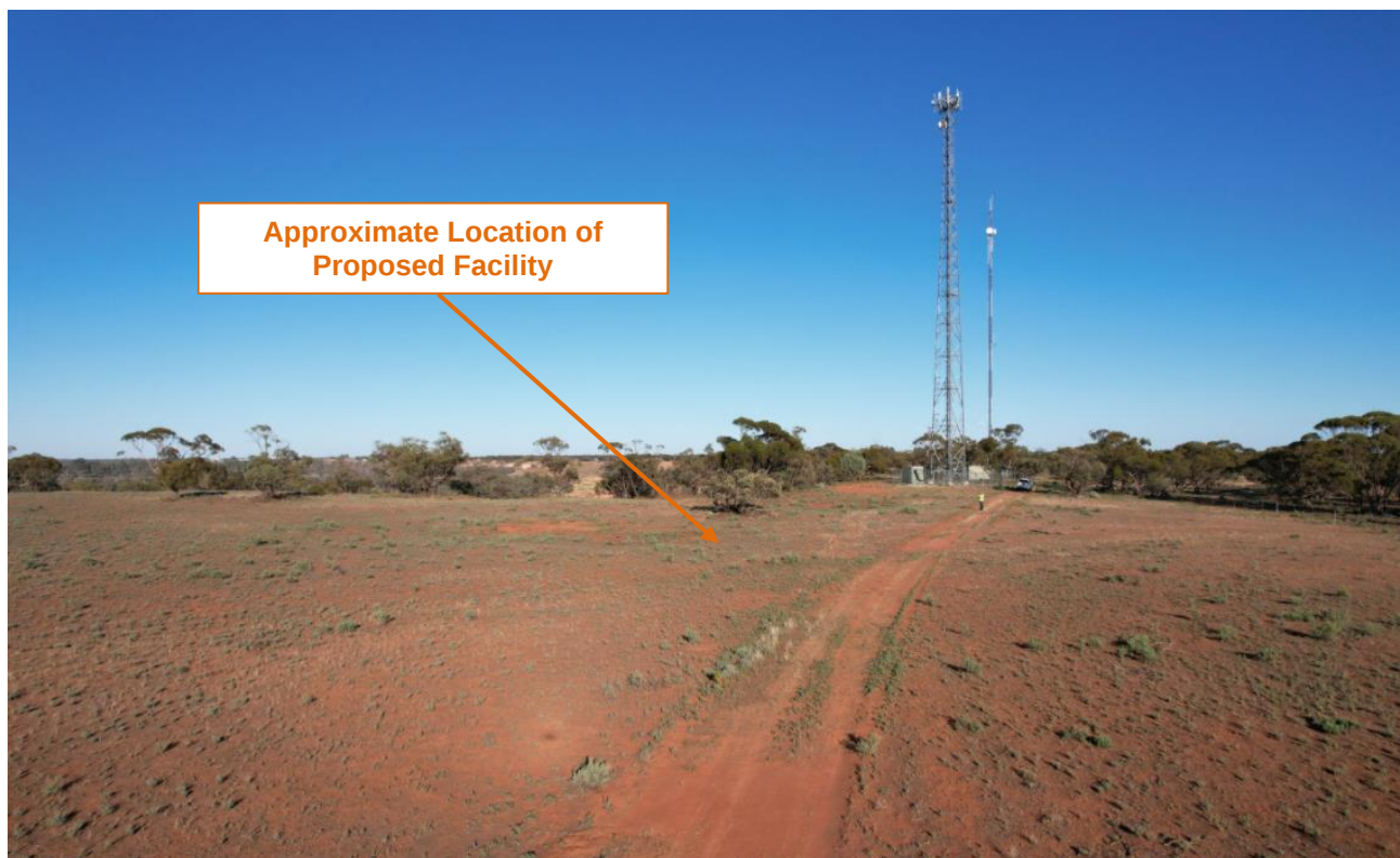
Figure 4: Proposed Telstra site location shown. Optus Lattice Tower (left) and Sydney Water guyed mast (right) in the background. Source: Servicestream, 3/2/22
